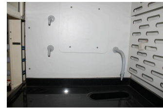
WATER TAP & SINK WITH DRAINAGE SYSTEM
